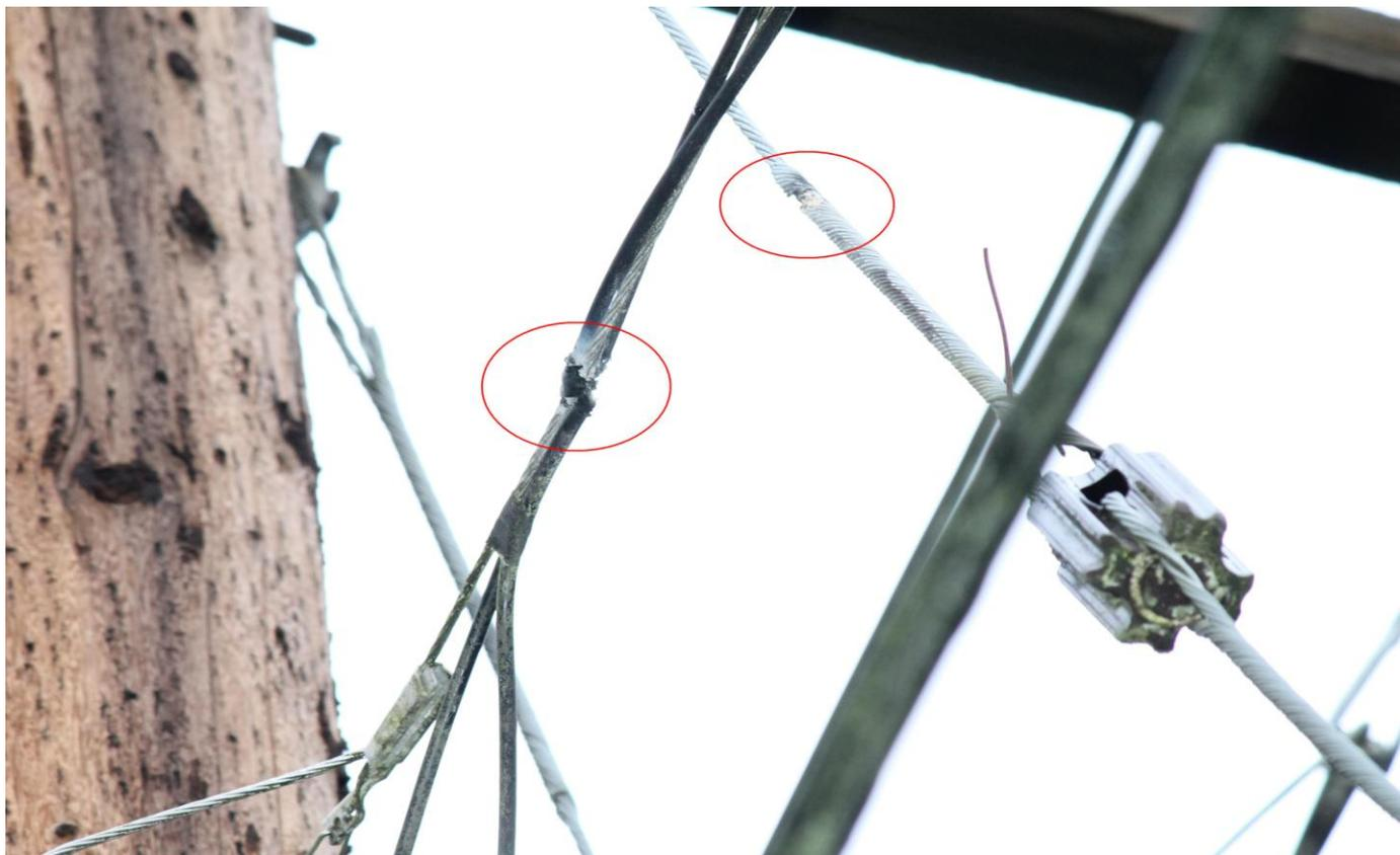
If there wasn't an insulator just inches under the contact point, the guy itself would be hot. I tied the guy wire so it came away from wire and took some pictures with a telephoto lens. As of a week later, it remains uncorrected but, at least, I know how to fix the noise.
